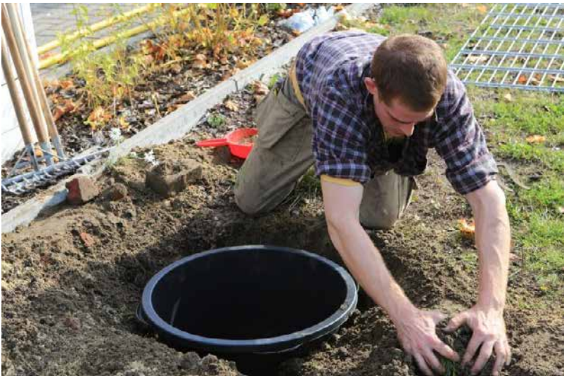
Completing the drainage pit
