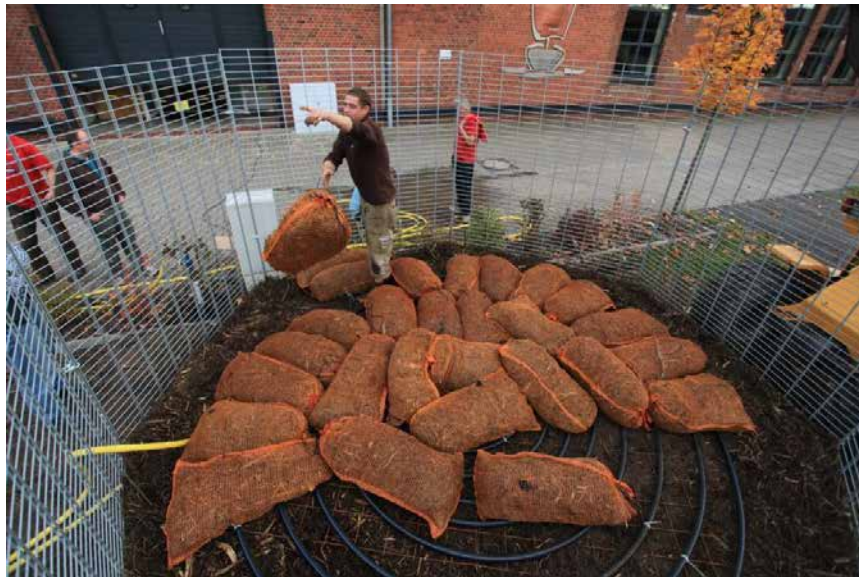
Covering the heat exchanger
