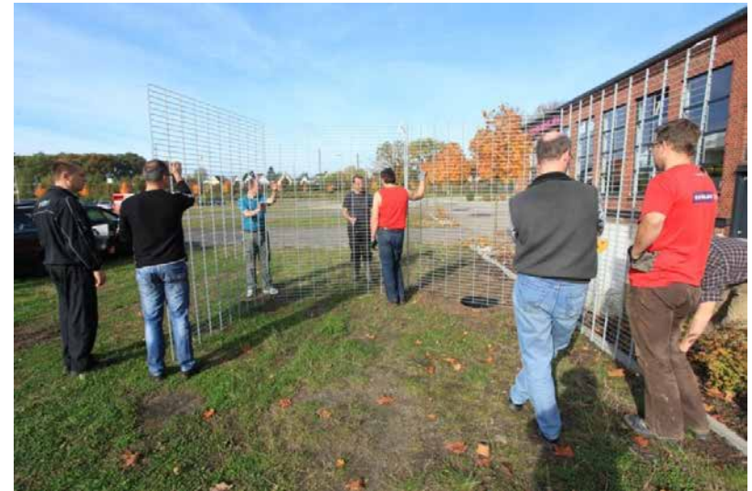
Allignment of fence elements
