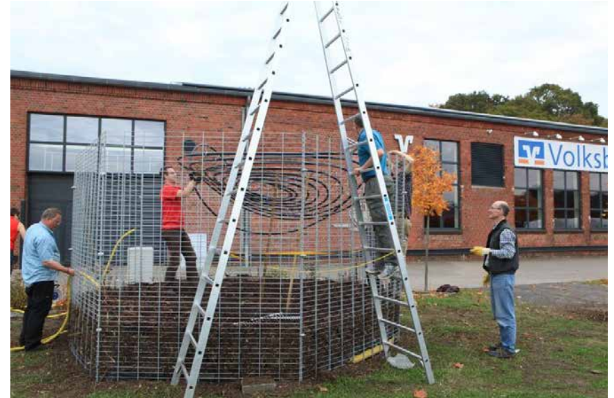
Applying the first heat exchanger
