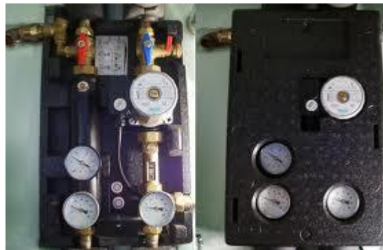
Thermic solar pump station
