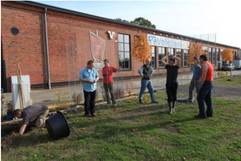
Set up of fence elements
